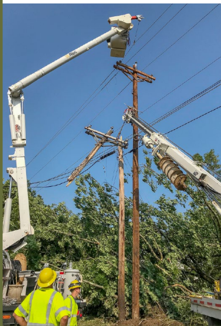
STORM DAMAGE. A Claverack line crew works to extract a broken pole top and cross arm that snapped off during an August storm in the Franklin Forks area. 2018 will be remembered as one of the wettest years on record in our region. The constant precipitation, often accompanied by high winds, caused flooding and tree-related outage problems throughout the year.
