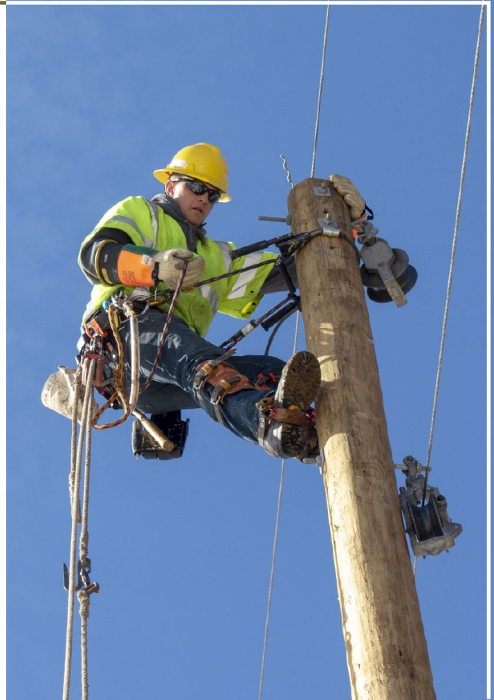
HIGH WIRE WORK. Apprentice lineman Troy Ely works on a system improvement project in the Montrose area in February.
