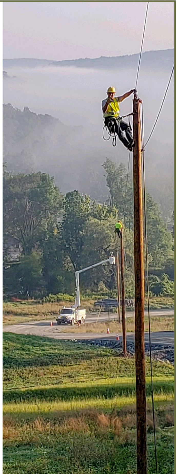
TEAMWORK. The Tunkhannock line crew builds a new section of line in the Lenox area on a warm summer morning in 2018.
